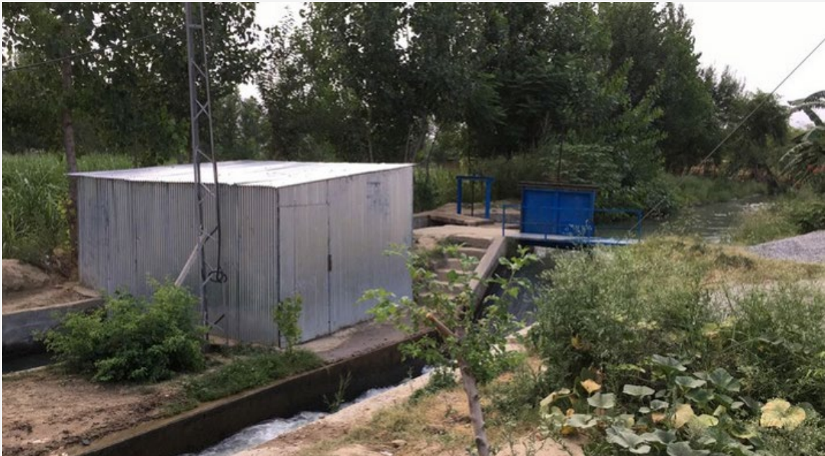
Microhydro generator installation at remote location (Sakhakot) in Northern Pakistan.
